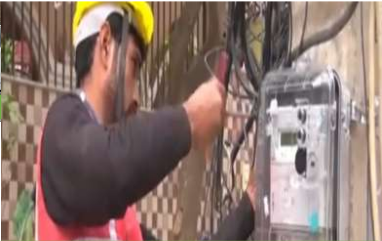
Quality & Safety Work and Trained Team
