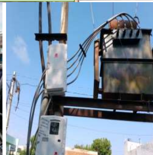
DT Meter Installation with Expert Team at Rajasthan
